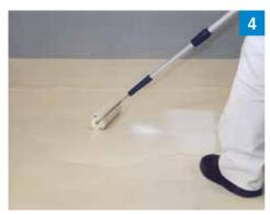
Apply the finish resin (without Triflex Liquid Thixo) to the surface and cross-coat by using a Triflex finish roller.
