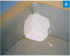
Then apply a thick layer of waterproofing resin on top of the inner corner fleece.
