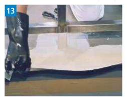
Use a roller to smooth out the fleece so that there are no air bubbles and apply another generous layer of waterproofing resin.
