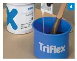
Add the appropriate weight of Triflex Catalyst and stir until there are no more lumps (see mixing instructions on the container).
