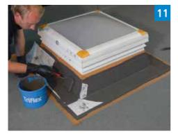
Then apply another thick layer of waterproofing resin to the fleece.
