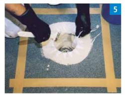
Apply a generous layer of waterproofing resin in and around the gully and lay the fleece cut-out for the gully, making sure there are no air bubbles.
