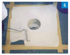
Apply a generous layer of waterproofing resin to the area in and around the gully.
