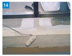
Finally, remove the adhesive tape from the leading edge while the resin is still wet.
