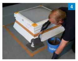
Then apply another thick layer of waterproofing resin to the outer corner fleece.
