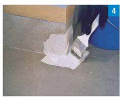
Then apply a thick layer of waterproofing resin on top of the outer corner fleece.
