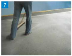
After the Triflex Cryl Finish 205 has cured (approx. 2 hours), carefully brush off any surplus Triflex Colour Mix. It is essential to ensure that the surface is kept free of any contaminants (e.g., dirty footwear, tools, etc.).
