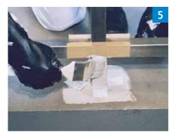
Apply another thick layer of waterproofing resin to the fleece.
