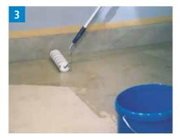
Apply primer to horizontal surfaces evenly with a universal roller to form a film layer.
