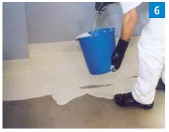
Apply the waterproofing resin for the second length of fleece and again spread it evenly.
