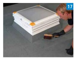
Once the resin has cured, remove any excess slate chippings.
