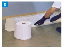
In the case of inner corners, lay the fleece approx. 5 cm around the corner and cut diagonally into the creased fleece on the floor right up to the corner.
