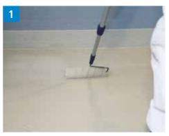
Dress the wet finish with plenty of quartz sand (grain size 0.2–0.6 mm).
