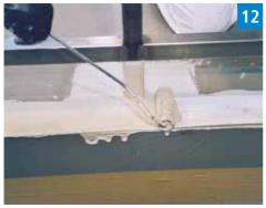
Apply a generous layer of waterproofing resin to the underside.
