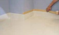
Important: In the case of vertical surfaces, add Triflex Liquid Thixo in order to make the finish thixotropic.
