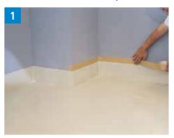
Important: In the case of vertical surfaces, add Triflex Liquid Thixo in order to make the finish thixotropic. Apply finish resin (incl. Triflex Liquid Thixo) to the vertical areas using a radiator roller or brush.
