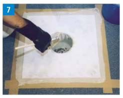
Lay fleece for the surrounding area, making sure there are no air bubbles, and use a brush to place the star-shaped incisions in the gully.
