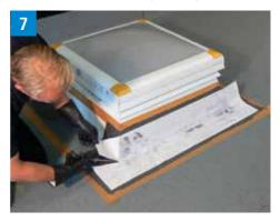
For the outer corners, the fleece is carried around the corner at least 5 cm and the fleece on the floor diagonally cut into up to the corner.
