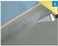
Use a funnel spray gun with special attachment to apply a generous layer of Triflex Colour Mix to the still-wet finish.
