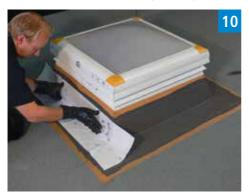
Lay the fleece cut-out for the surrounding area making sure that there are no air bubbles, cut into the fleece diagonally and lay around the corners.
