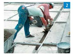
After priming, fill any repair points and areas of damage with mortar.
