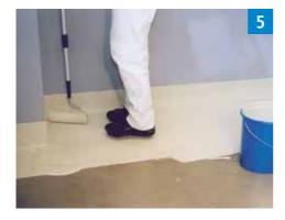
Remove any air bubbles by working the roller out towards the side.
