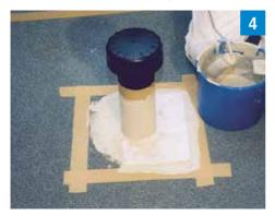
Apply waterproofing resin to the surrounding surface area, lay the first surface fleece cut-out, making sure there are no air bubbles, and apply another generous coat of resin.
