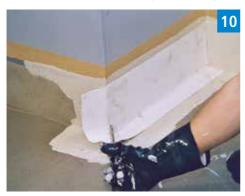
In the case of outer corners, lay the fleece around the corner approx. 5 cm and then cut diagonally into the fleece on the floor up to the corner.
