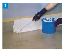
Either pre-cut the Triflex Special Fleece or apply straight from the roll onto the fresh resin ensuring there are no air bubbles. Make sure the fleece is fully saturated.
