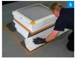
Lay the fleece cut-out for the surrounding area making sure that there are no air bubbles.
