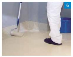
Apply finish resin (without Triflex Liquid Thixo) to floor areas by using a Triflex finish roller.
