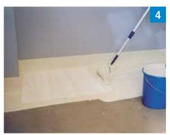
Cover the laid fleece with enough resin – wet on wet – to ensure full saturation.
