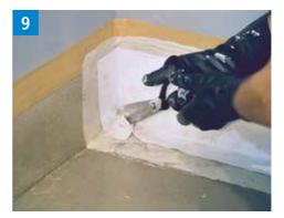
Important: To ensure proper saturation of the fleece, this initial coating should be applied to no more than 2 meters at a time. Then lay the fleece and apply another generous coating immediately.
