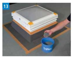
If the waterproofing needs to match the surrounding area, the surface can be dressed with slate chippings.
