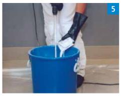
Add the Triflex Catalyst to the running mixing machine until there are no more lumps (see mixing instructions on the container).
