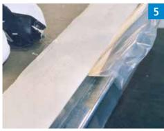
Remove the adhesive tape and sheet while the resin is still wet.
