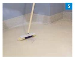
Remove the excess Triflex Micro Chips before applying the surface finish.
