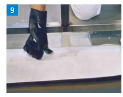
Lay cut sections or rolled strips of fleece so that there are no air bubbles and paying attention to the depth of the flashing at the leading edge.
