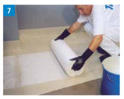
Cover the fleece again with enough resin – wet on wet – to ensure full saturation.
