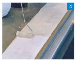
Then apply another thick layer of waterproofing resin to the fleece.
