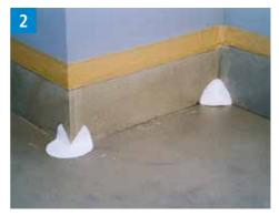
Important: A sufficient amount has been applied if the fleece is fully saturated. If the fleece is not fully saturated, lift it off and apply another generous coating.
