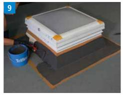
Apply a generous layer of waterproofing resin for the next partial area.
