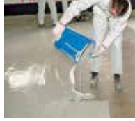
3. Triflex DeckFloor self-levelling mortar is applied ...
