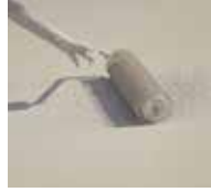
4. ... and spread evenly using the Triflex Special Roller.
