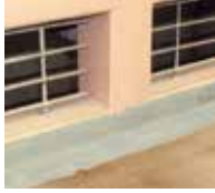
2. The details are waterproofed using Triflex ProDetail.
