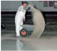
5. The wet coating can be sanded down, e.g. for parking bays.
