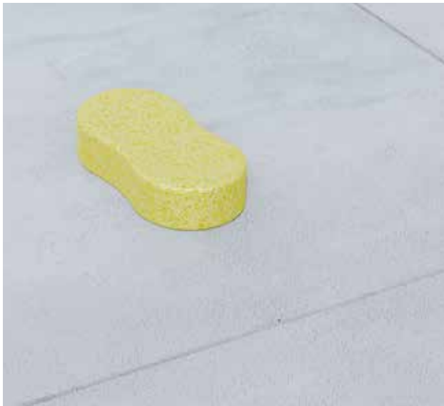
Clean and degrease the surface
